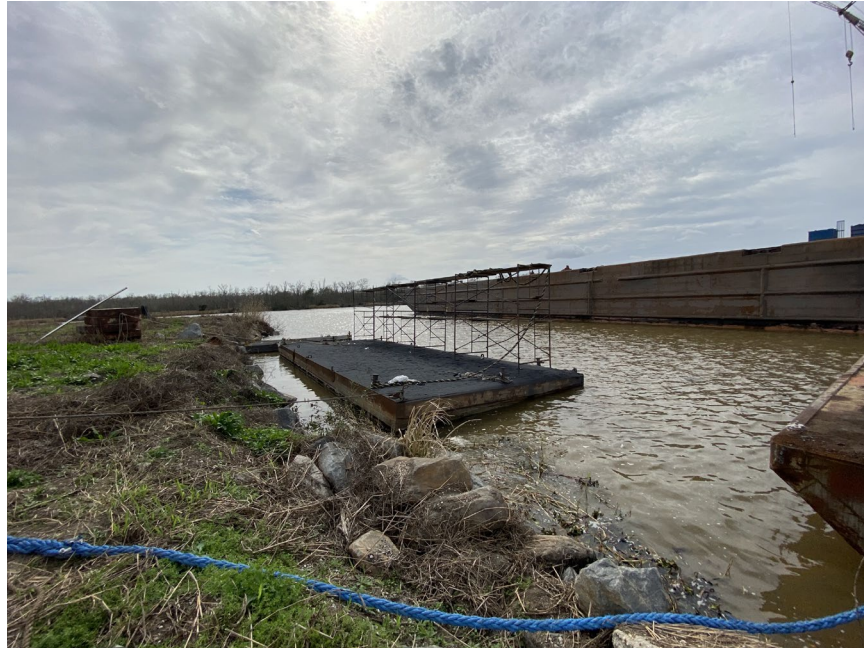
Photograph of small work barge with scaffolding adjacent to the side hull of the freight barge.
